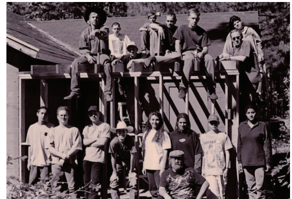
Construction Class, circa 1983
