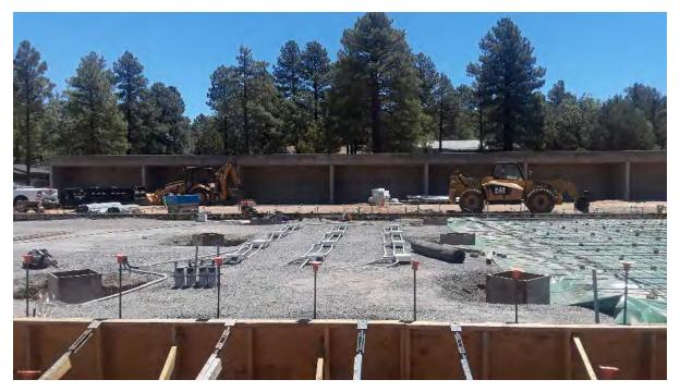
View is looking to the southeast showing the floor in the EIT and Welding Shop portion of building #1, ready to receive concrete. The structural steel of building #3-Automotive Shop is in the background. Storage bunkers are to the left. Concrete form edge panels and bracing are in the foreground.
