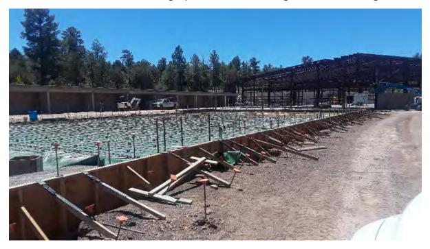
This view is looking south into the project from the future north parking lot. One of the concrete retaining walls is on the right of the picture. Rip-Rap stone has been placed part of the wash (on right). Workmen are finishing the plumbing, electrical floor boxes, and electrical conduit under the floor slab. Concrete edge forms and bracing. Structural steel of the Automotive Shop is in the background.
