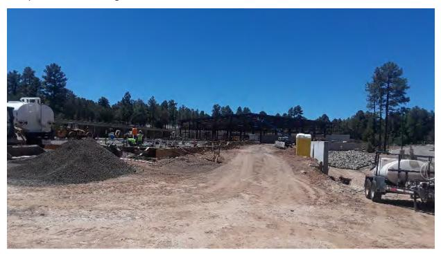
Student Commons restroom/locker room slab with plumbing drains and vent risers exposed. IT room in back righ hand side of Commons slab. Structural steel of Automotive shop on right. Bunkers in the background. Edge forms and reinforcing steel of Welding shop on the left.
