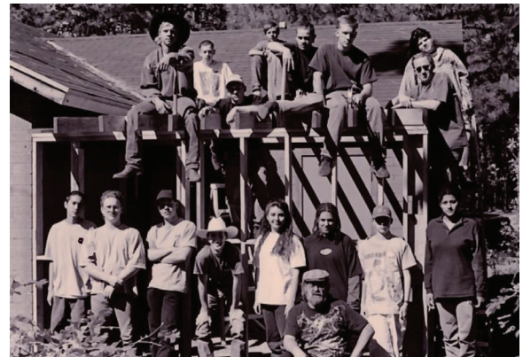
Construction Class, circa 1983
